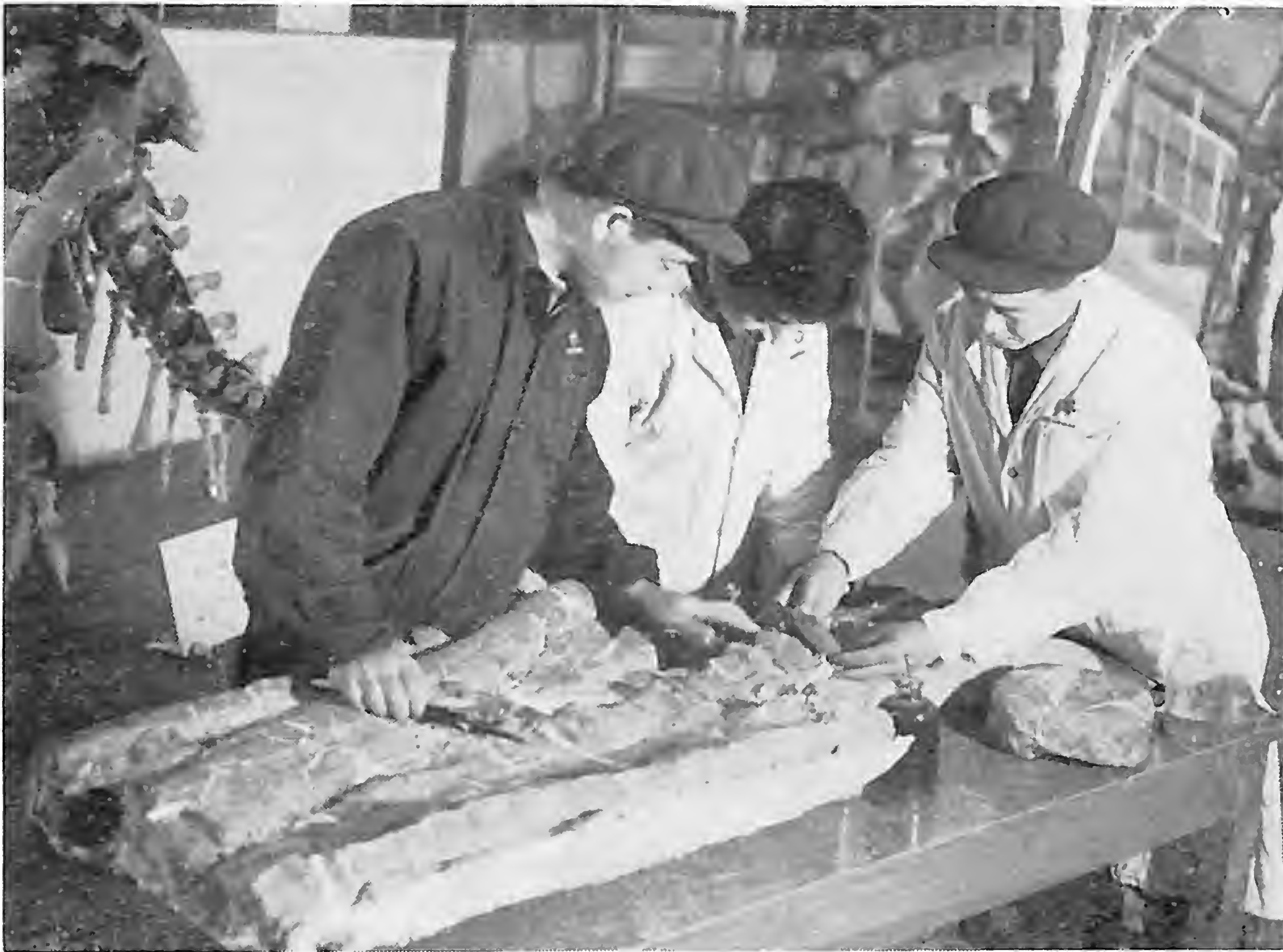
Discussing restoration and reconstruction.
